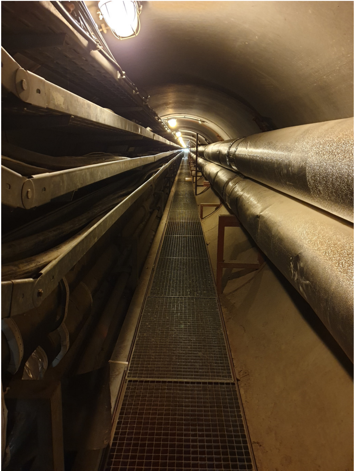
Figure 2.2: Example of a collector shaft.
