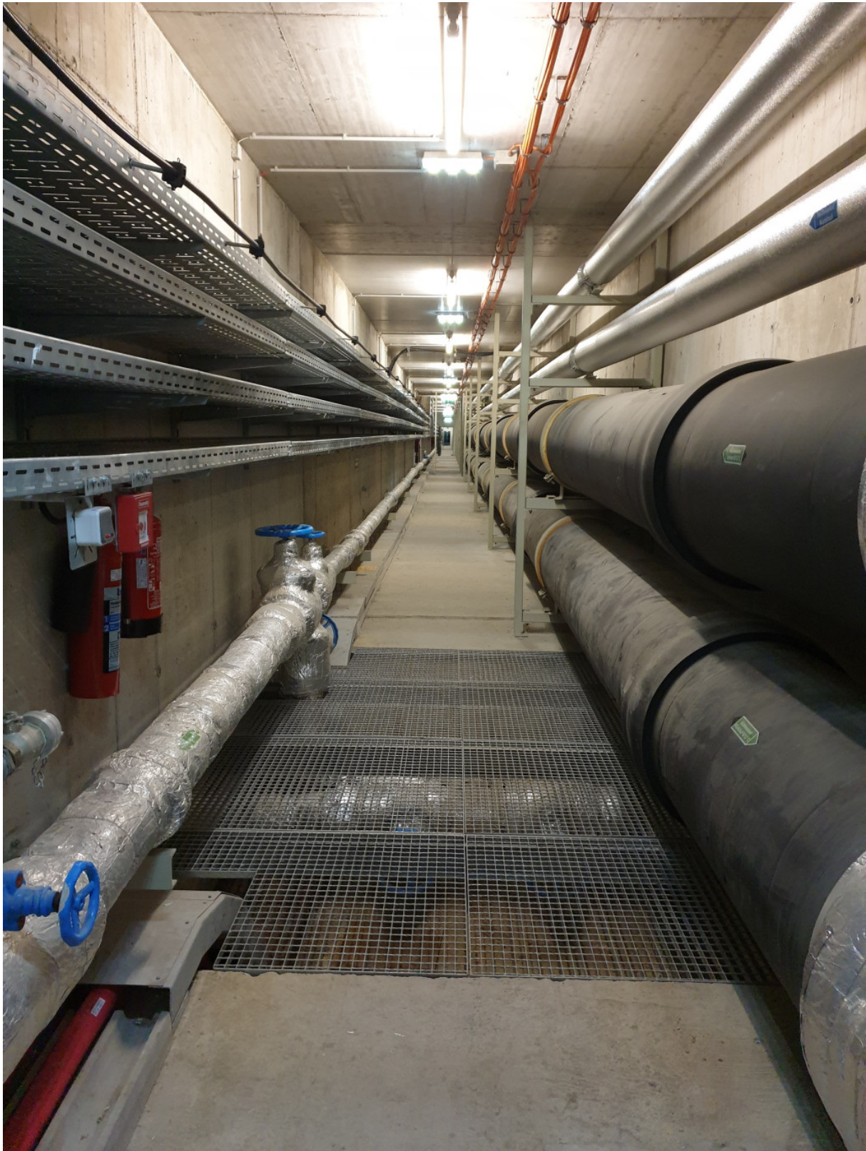
Figure 2.1: Example of a collector shaft.
